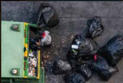
Waste Removal & Site Clean-Up
